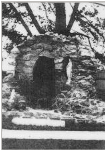
This commemorative grotto was constructed at the Presentation Convent in 1937 to mark 25 years since the arrival of the first three Sisters in 1912. It was built by former student Ted Green with stone supplied by another past student, Bernie Leigh.
