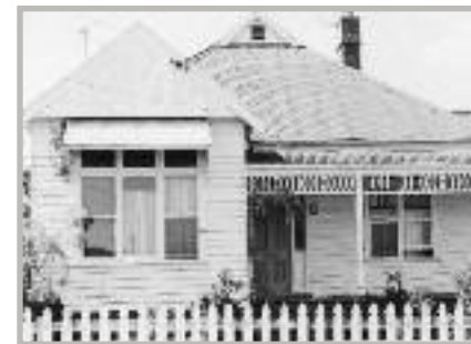
The house at 75 Langhorne Street was purchased in 1969 to house the growing Presentation community.
